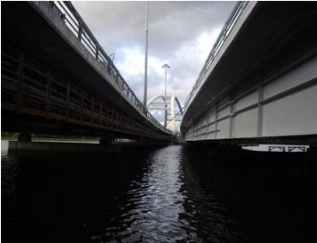
Bridge over the Okhta River, constructed during 2004 – 2008. Part of the ring road around Saint Petersburg. Length 333.7m. Painted area of 250 000m<sup>2</sup>. Paintwork performed in accordance with the Russian standard for bridges, STO-001-2006.
