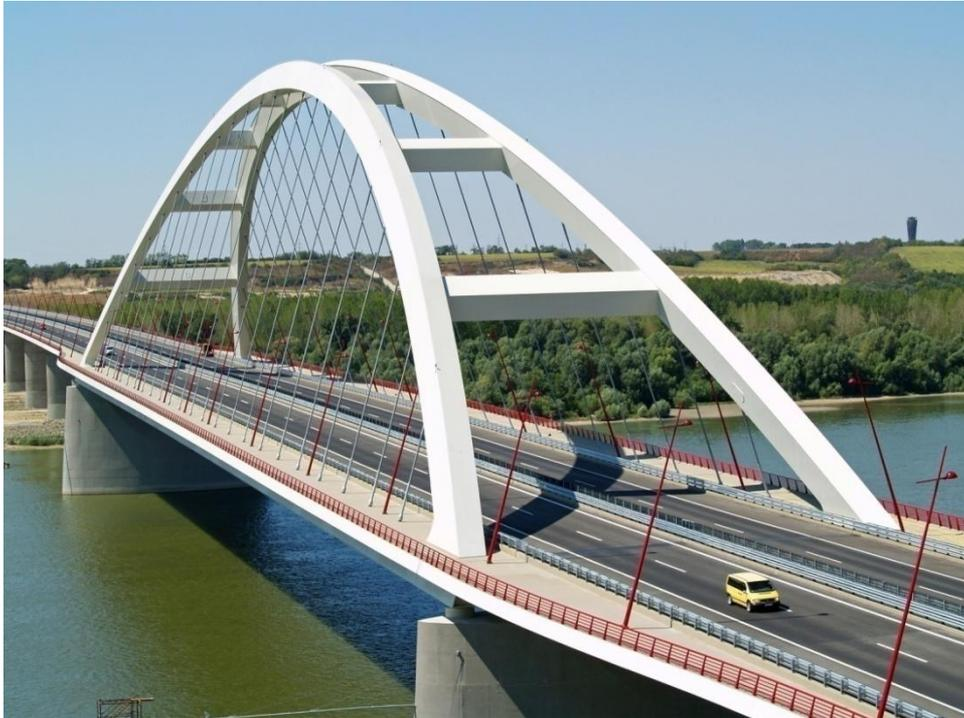
One of the biggest public bridges in Central-Eastern Europe. Length 1677 m and width 32.3 m. Constructed in 2007 with 24 000 tons of steel structures.
